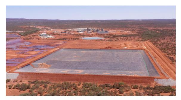
Figure 8 – Completed TSF in the foreground with processing plant and box-cut in the background (Photo 14 October).
