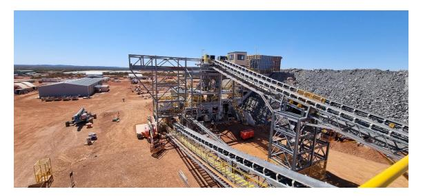
Figure 6 – Abra crushing and screening area to commence dry commissioning in October. Site stores and plant workshop building seen on the left (Photo 14 October).
