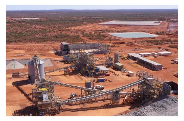
Figure 1 - Processing plant with completed TSF and village in background (Photo 14 October).
