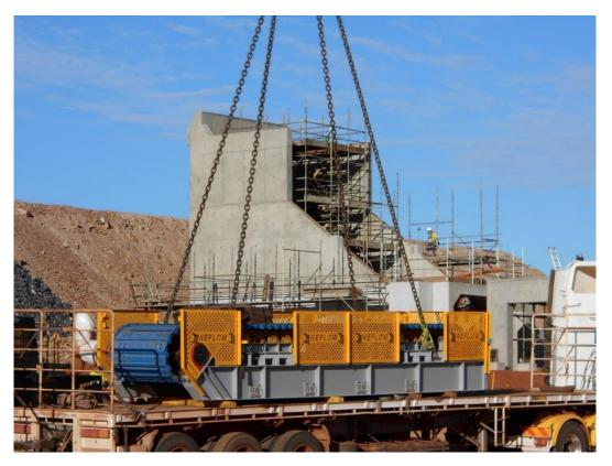
Figure 6 – Arrival of primary crusher feeder.
