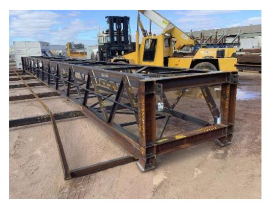
Figure 9 – Conveyor truss fabrication in Perth.
