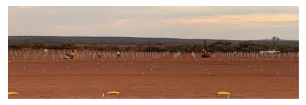
Figure 13 – Post-hole drilling and piling prior to commencement of solar panel installation.
