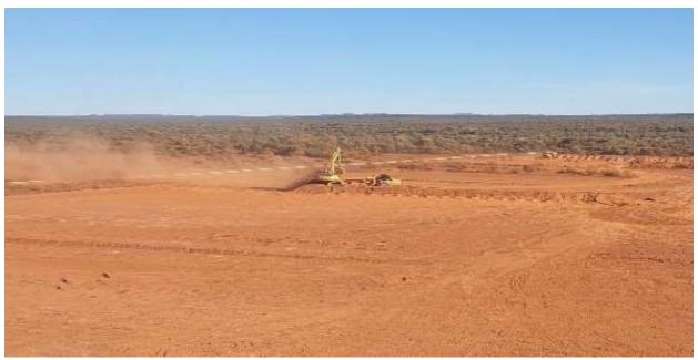
Figure 3. Load and haul of topsoil at site of future processing plant.
