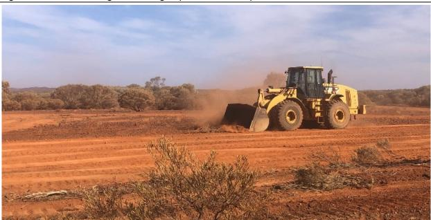
Figure 1: Loader working on clearing at permanent camp site
