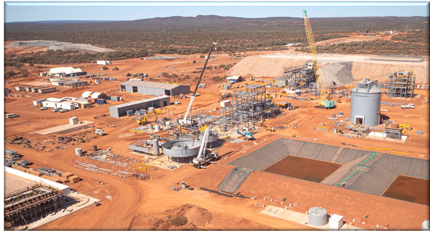
Processing Plant Construction - July 2022
