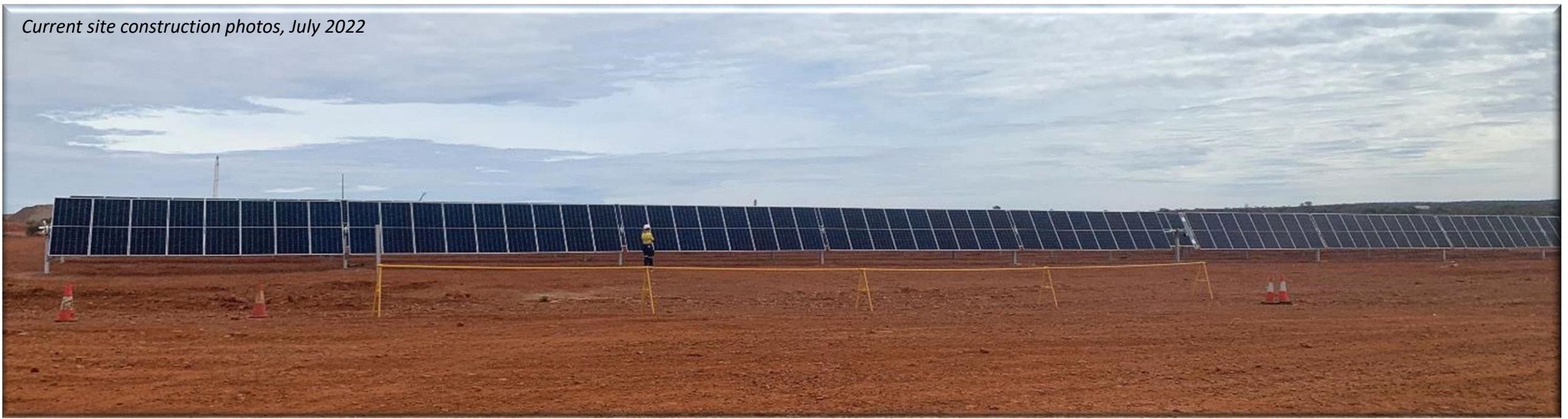
16,000 solar panels installed
