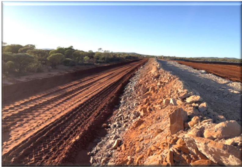
TSF – under construction
