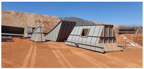
Figure 4 – Crusher chutes and bins on site ready for installation.
