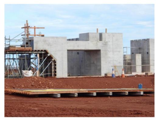
Figure 6. Grinding mill plinths.
