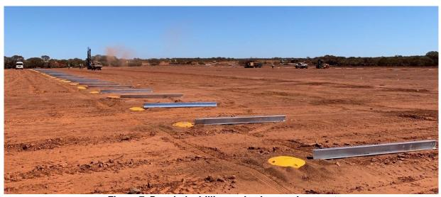
Figure 7. Post-hole drilling and solar panel supports.
