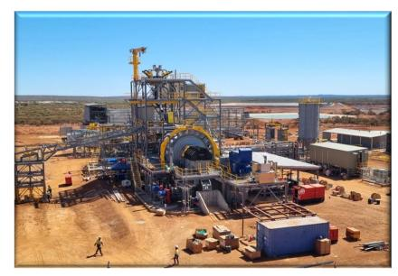
Grinding, Flotation & Filtering Sections
