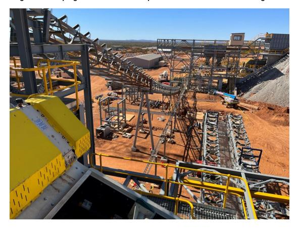
Figure 5. Crusher area with commencement of conveyor installation (July Photo).
