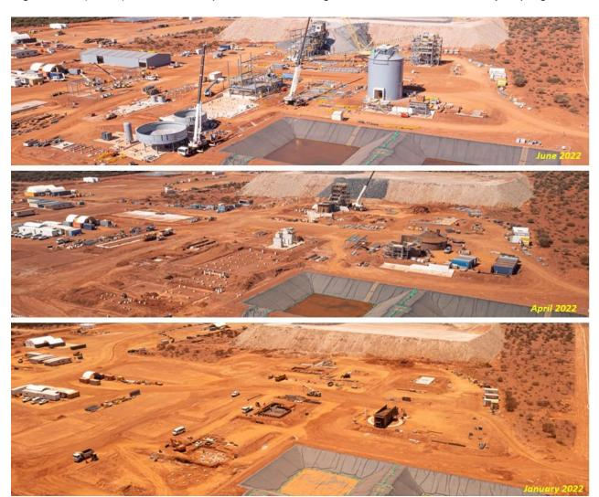
Figure 3. Work progress from January 2022, through April 2022 to June 2022 at the main Abra plant and infrastructure area looking South.
