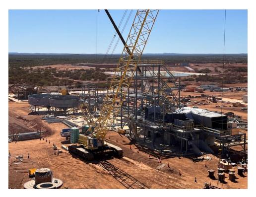
Figure 6. Processing plant construction, mill, flotation, thickening and concentrate sections (July Photo).
