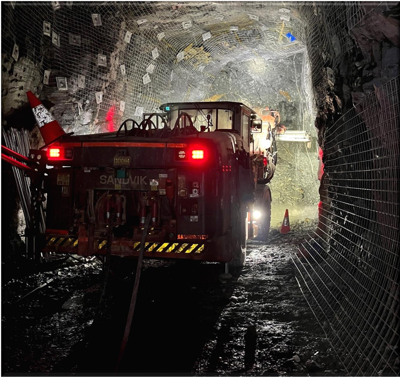
Underground Decline Development
