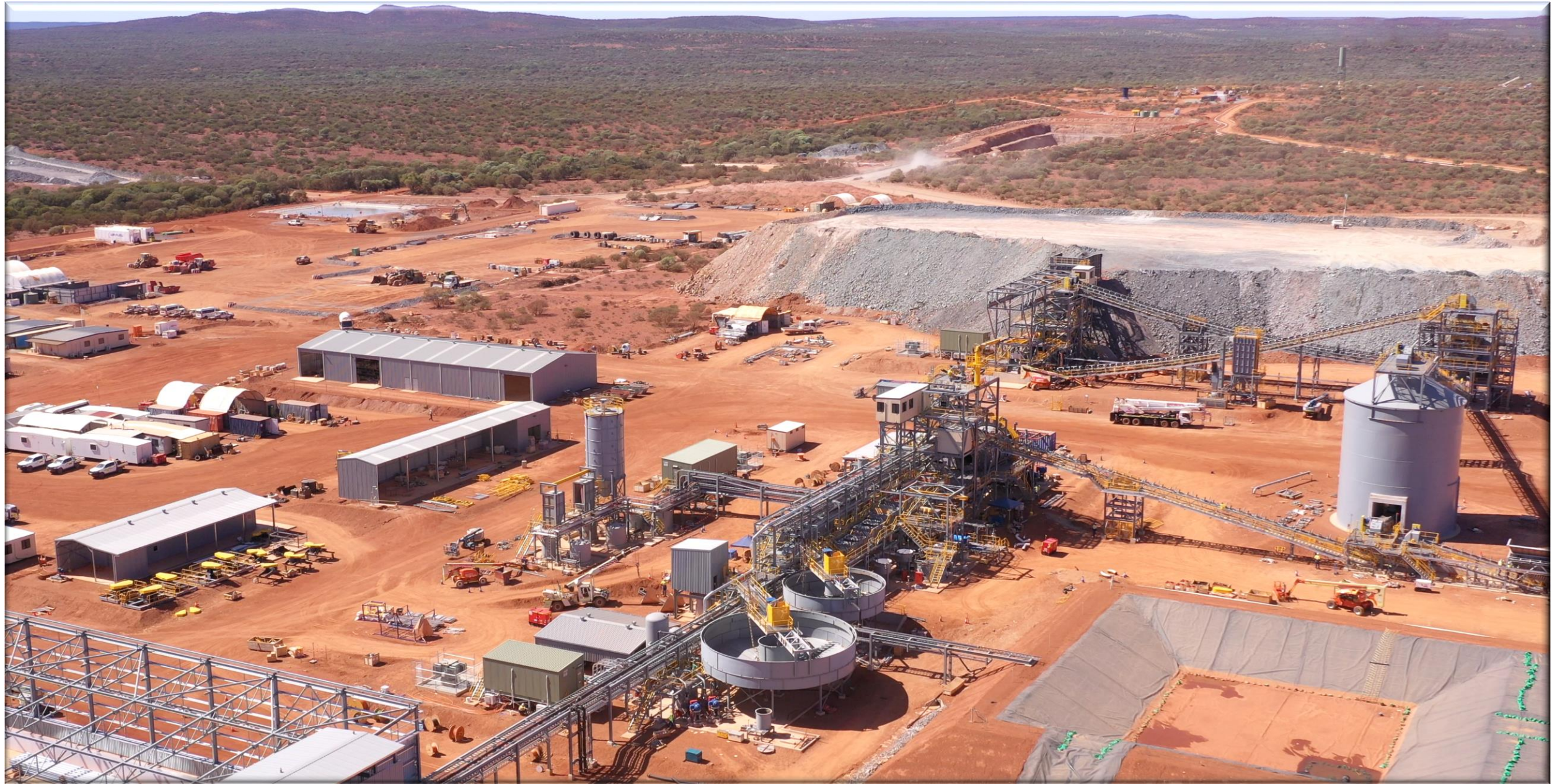
Processing Plant & Boxcut, October 2022
