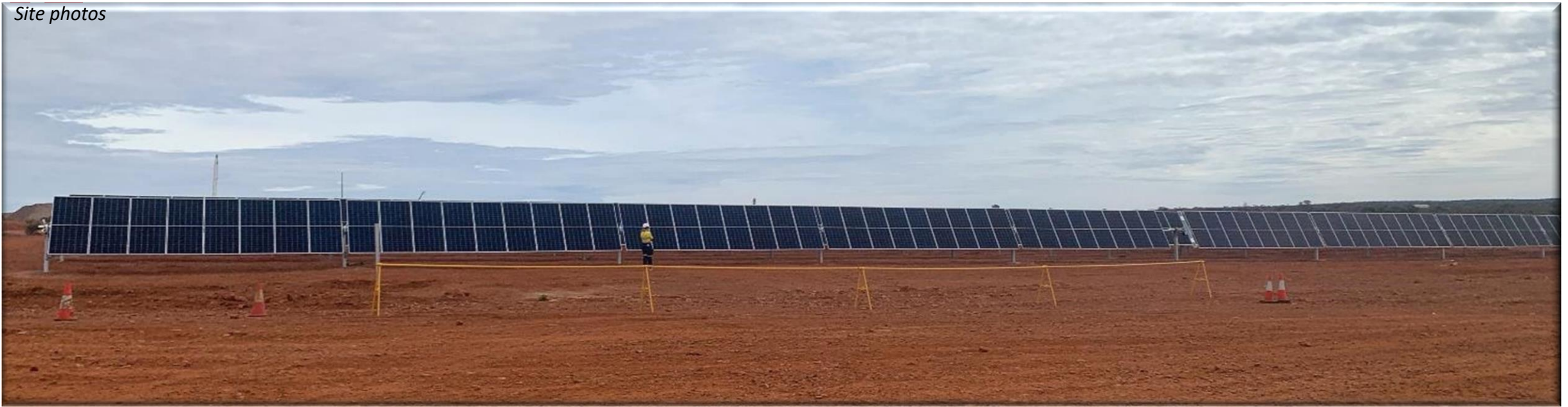
16,000 solar panels installed
