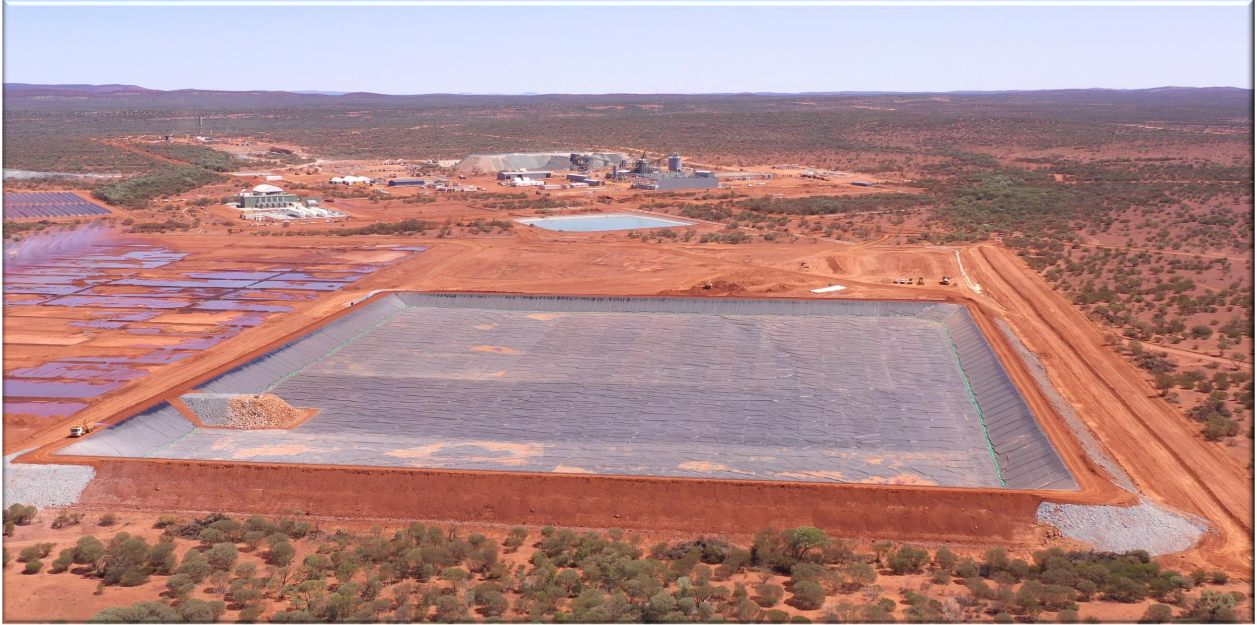
TSF, Power Station & Processing Plant, October 2022
