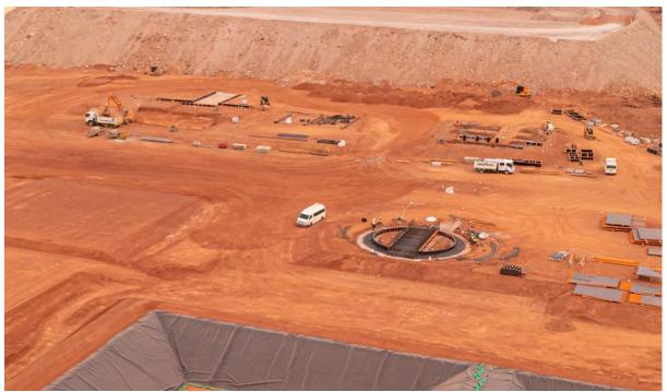
**Figure 2** – Civil construction progress with crushing/screening plant foundations. Completed raw and freshwater dams in the foreground.
