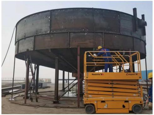
Figure 6 – Concentrate thickener fabrication.
