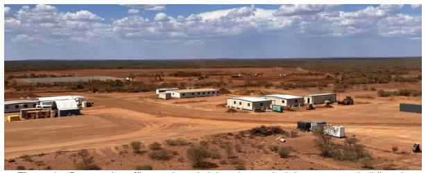
**Figure 4** – Construction offices, mine administration, and mining contractor buildings in place. Completed plant site earthworks in the foreground and civil construction occurring in the background on site power station earthworks.
