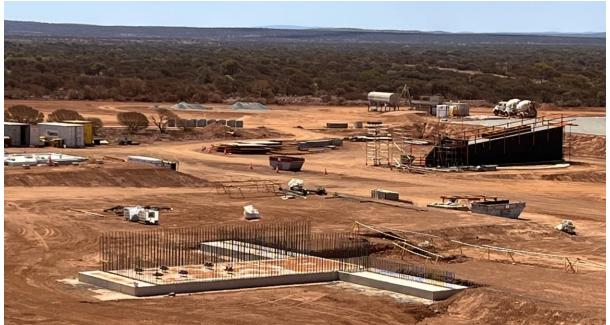
**Figure 7** – Processing plant site works showing crusher, screening, and ore storage foundations.
