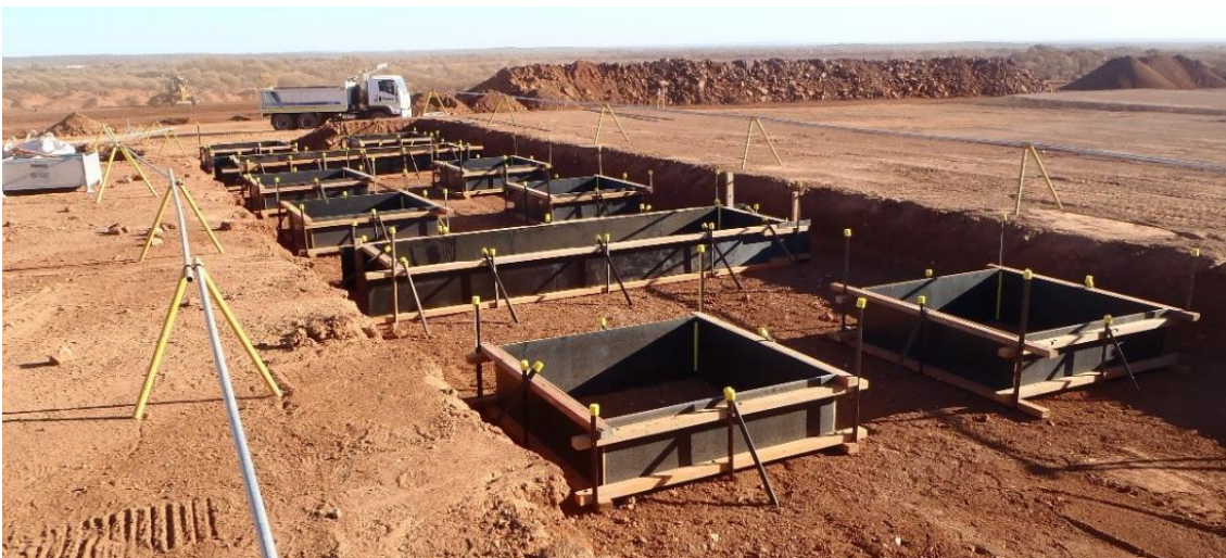
Figure 5. Processing plant (flotation area foundations).
