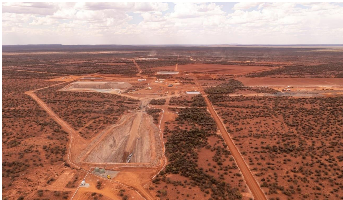
Figure 2. Aerial view of Abra (above the boxcut looking north towards the ROM pad and processing plant site in the middle ground, with the 280-unit accommodation village in the background).
