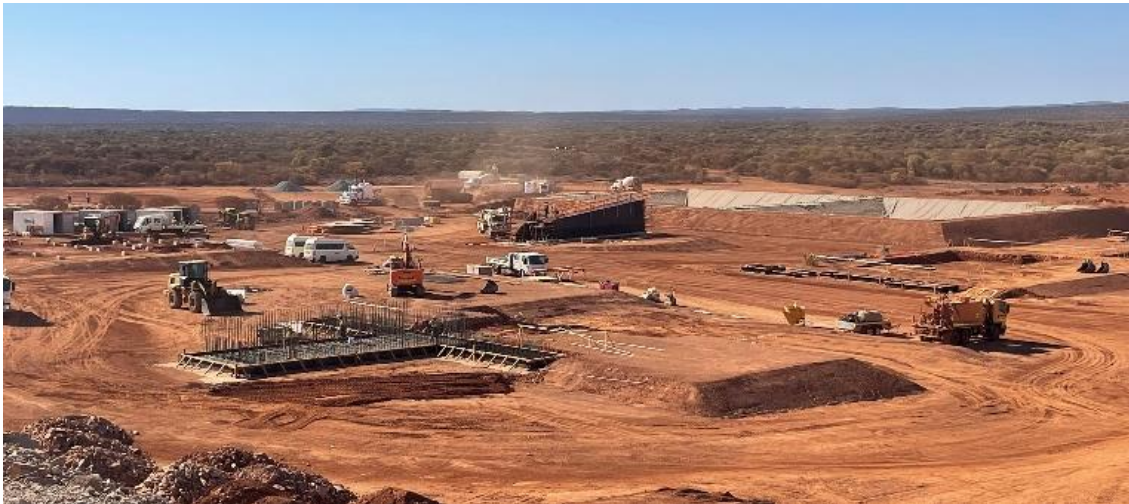
Figure 3. Processing plant civil and concrete construction in December 2021.
