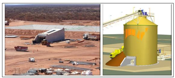
Figure 4 – Fine ore bin (FOB) concrete vault on the left with the design model of the FOB shown on the right.
