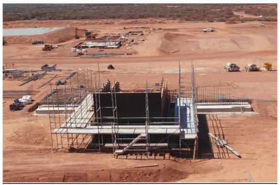
Figure 3 – Crusher wall formwork in the foreground and the mill concrete foundations in the background.
