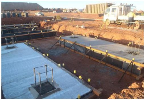
Figure 5 – Flotation area concrete footings.
