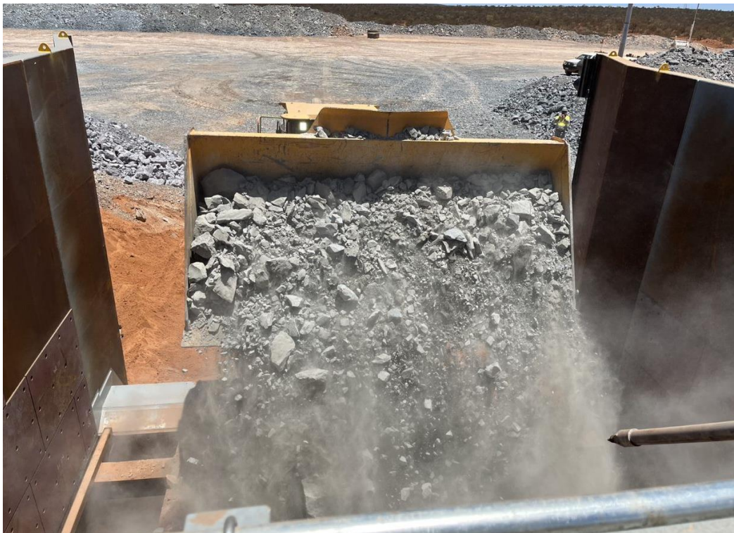
Figure 1 – First material being tipped into the crusher during commissioning (Photo 26 November).
