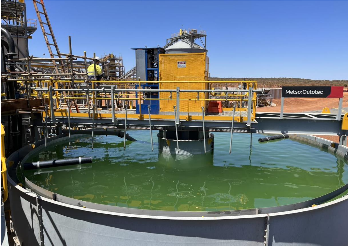
Figure 12 – Concentrate thickener full of water.
