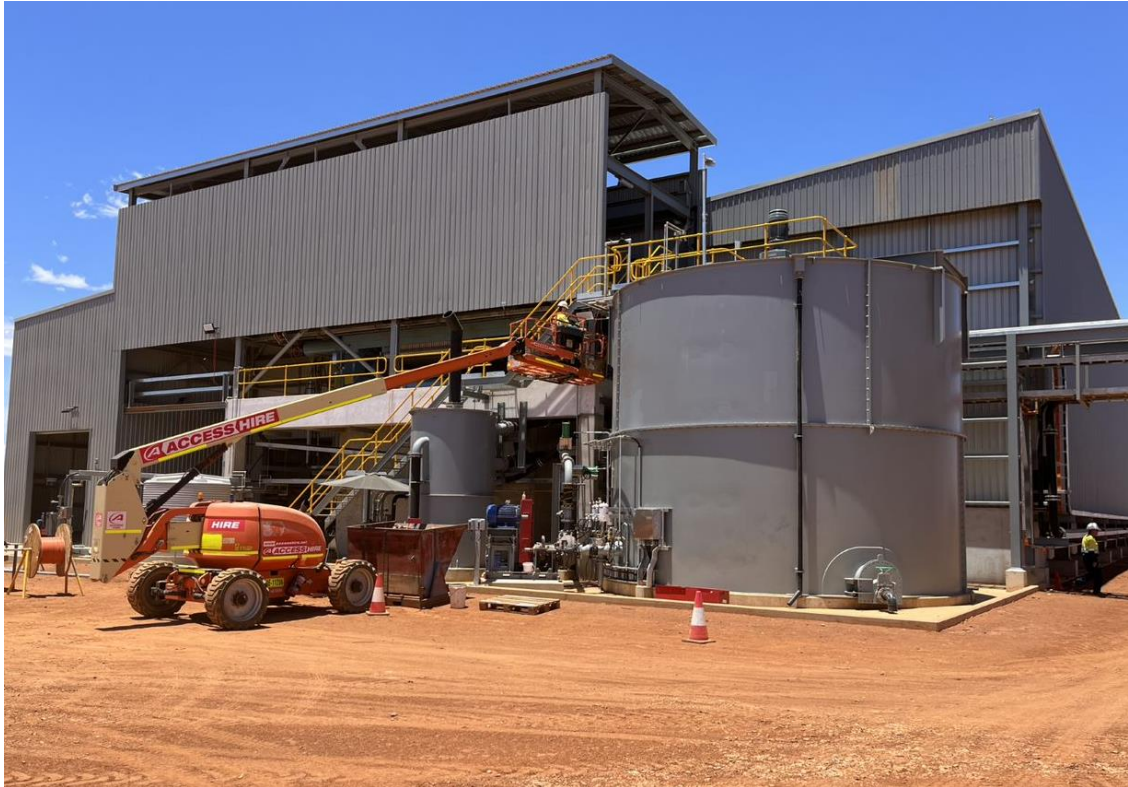
Figure 18 – Concentrate shed tank wiring installation.
