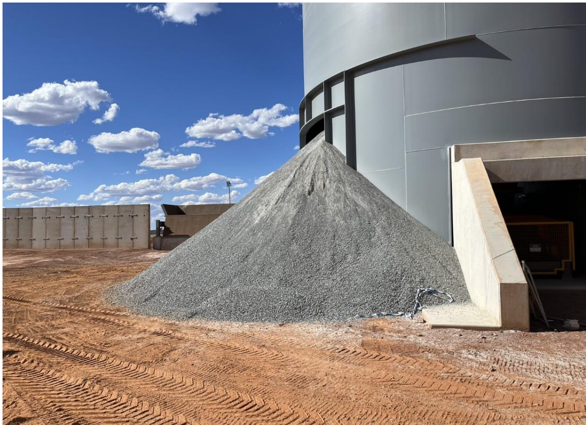
Figure 9 – Fine ore bin filled with inert waste.
