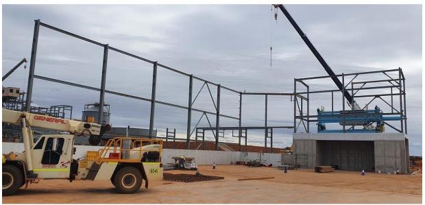
Figure 11 - Concentrate filter and shed construction.
