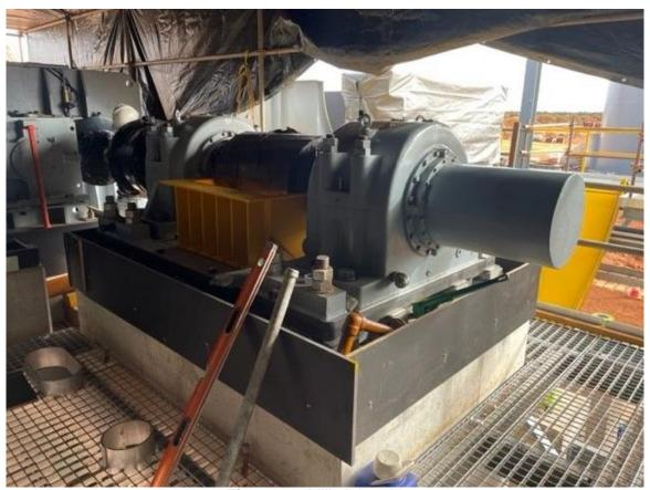
Figure 7 – Mill pinion drive.
