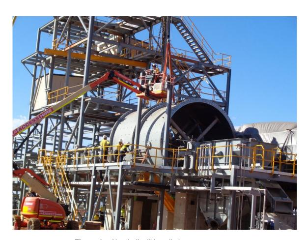
Figure 1 – Abra ball mill installation (photo: 10 August).
